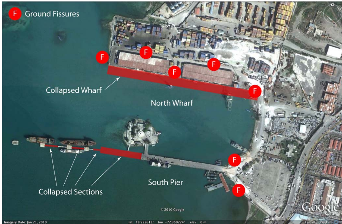
Figure 6.5 Annotated aerial image of Port de Port-au-Prince showing locations of damage due to the earthquake. Imagery courtesy of Google Earth. (N18.555058°, W72.351144°)
