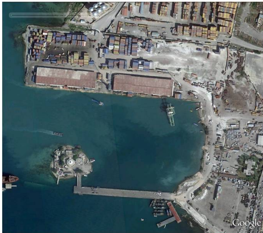
Figure 6.2 Pre- and post-earthquake satellite/aerial imagery (top and bottom, respectively) of the port at Port-au-Prince, Haiti (N18.555058°, W72.351144°). Imagery courtesy of Google Earth.
