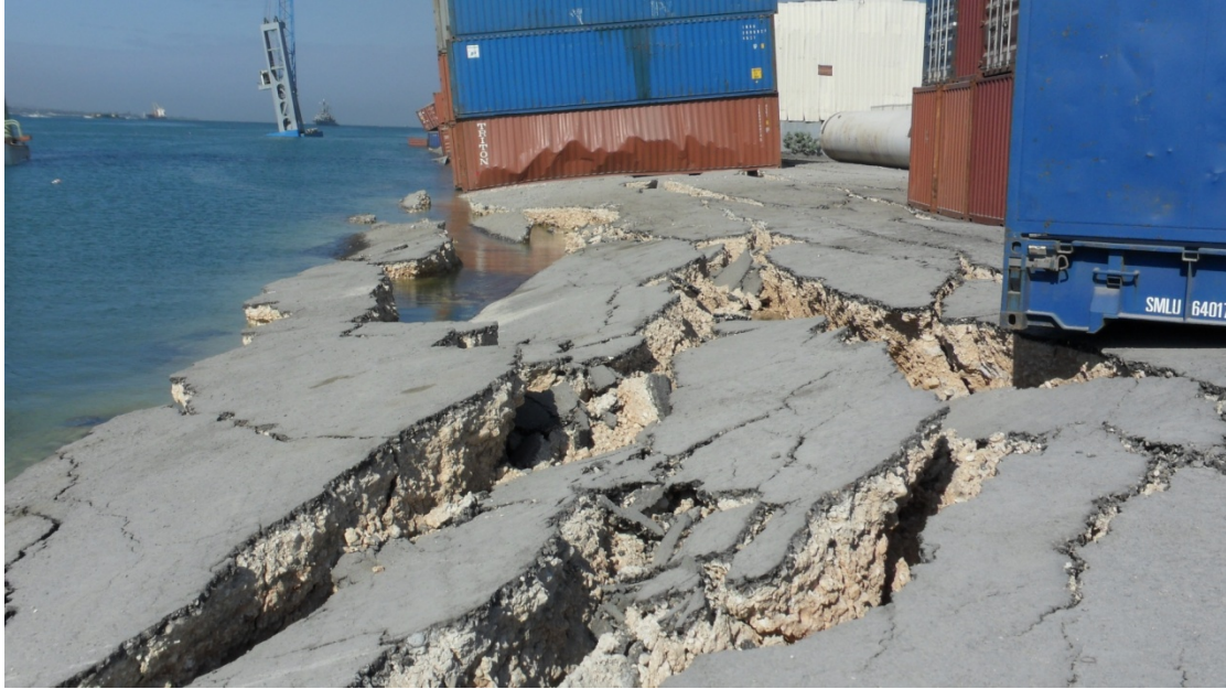
Figure 6.6 Lateral spreading adjacent to the collapsed North wharf. Note the crane in the water in the background and the metal warehouses on the right. (N18.55622, W72.34787)
