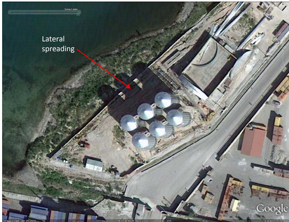
Figure 6.18 Lateral spreading behind (westward side) steel grain hopper silos. However, the foundation system for the silos showed no visible signs of distress. Imagery courtesy of Google Earth.
